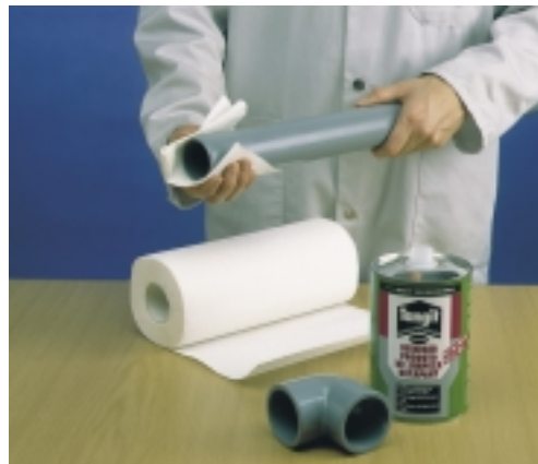
Cleaning the pipe and socket
