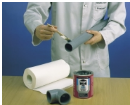
Applying the cement
