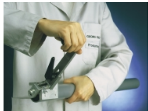
Chamfering the pipe
